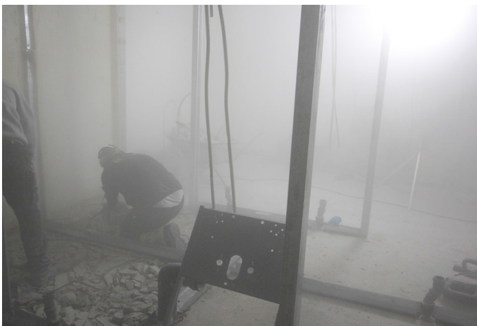
The dust situation when the room is removed from construction waste.
